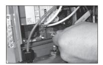
Attach the black wires from the Heat Pump Relay Kit to the main circuit board using the tabs near the heater terminals.
